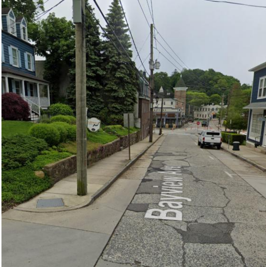
Bayview Avenue (Narrow sidewalk & non-compliant curb ramps)
